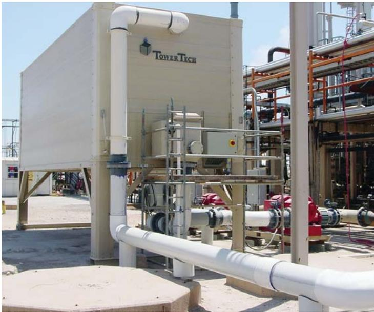
of temporary units. To enhance durability, reduce weight, improve longevity and aesthetics, and to increase protection against corrosion and fiber blooming caused by ultra violet light, wall construction was changed to heavy-duty continuously pultruded reinforced fiberglass containing premium isophalic resin in 1994. This change allowed Tower Tech to begin mass-producing Modular Cooling Towers.
